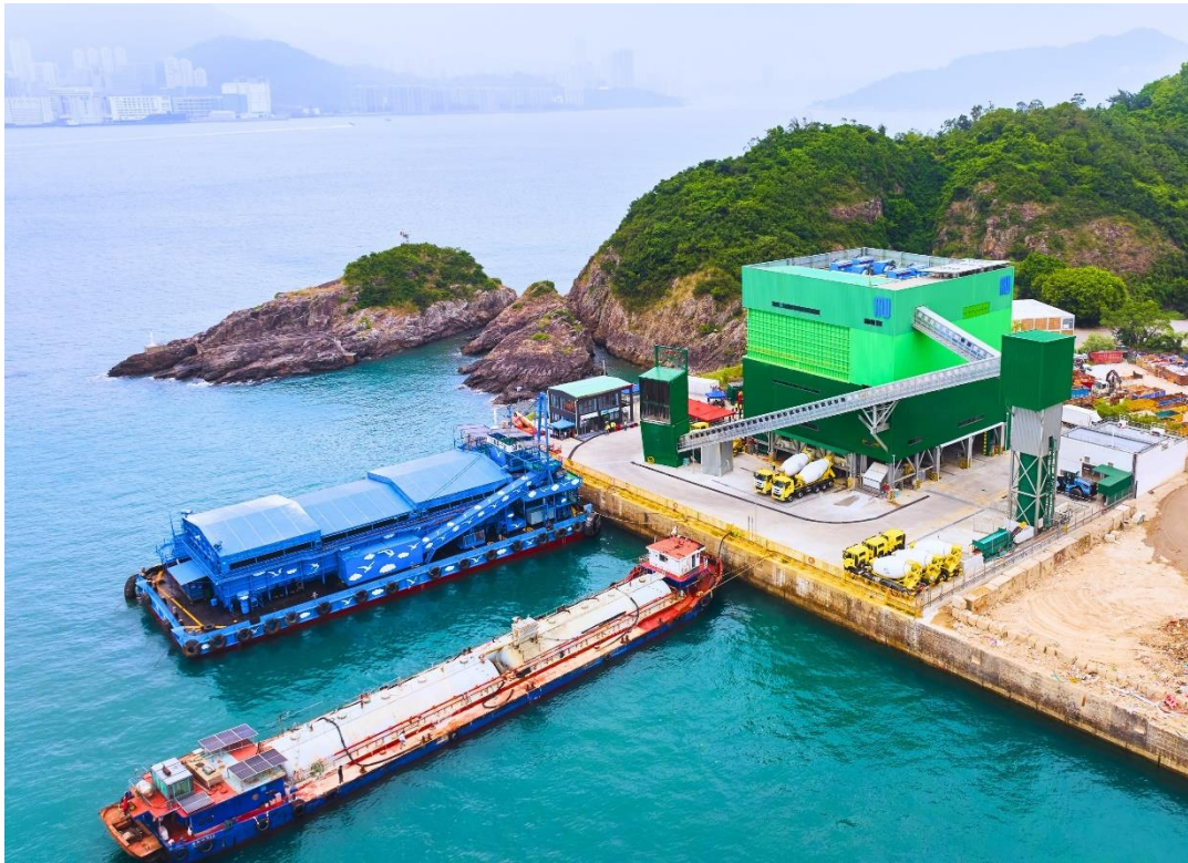
Tseung Kwan O Area 137 Concrete Batching Plant
