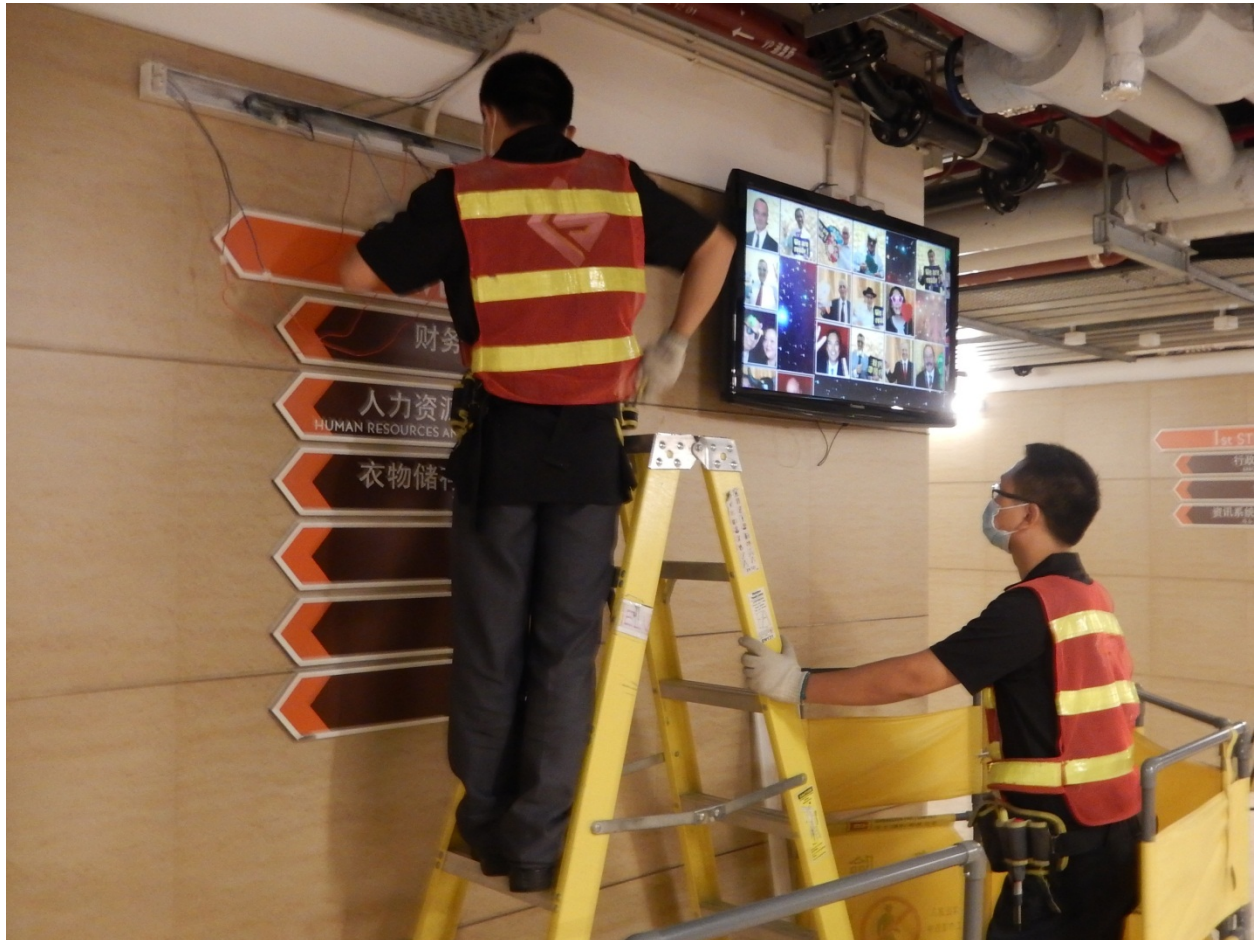
P002: GEG properties and their back of the house had changed to LED lights for energy saving.
