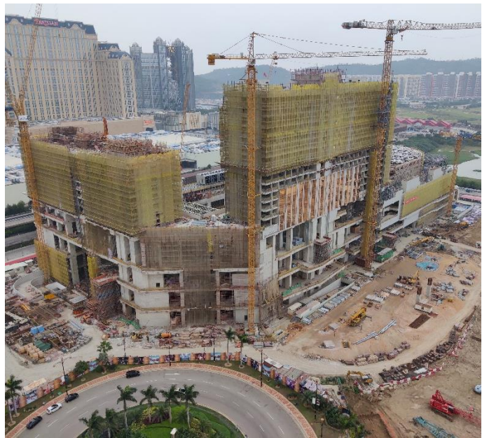
Photographs of Phase 3 development as at February 2020. The buildings have been topped out and we are commencing external cladding and internal fit out.
